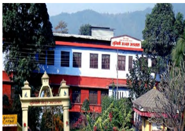
Lumbini District Hospital
